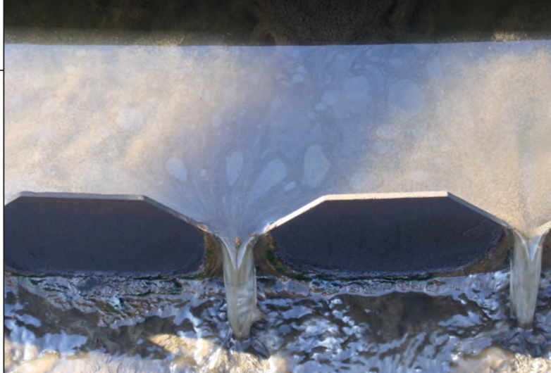
FIGURE 2. This photo depicts the clarification step of the activated sludge process
